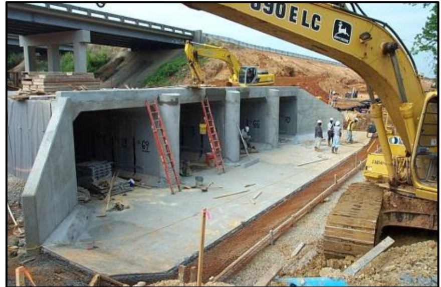
I-20 Bridge Replacement – GDOT Quad 12'x10' Bridge Replacement
